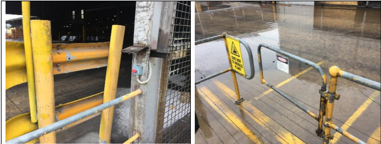
Figure 6: Manual Gate to Separate Pedestrian and Mobile Plant.
