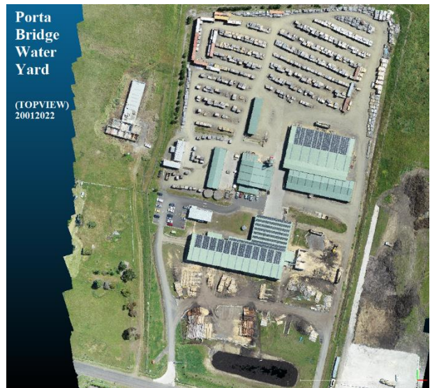
Porta Mouldings Bridgewater drying yard
