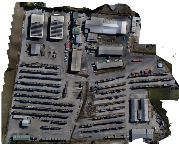
Britton Timbers' Smithton West drying yard
