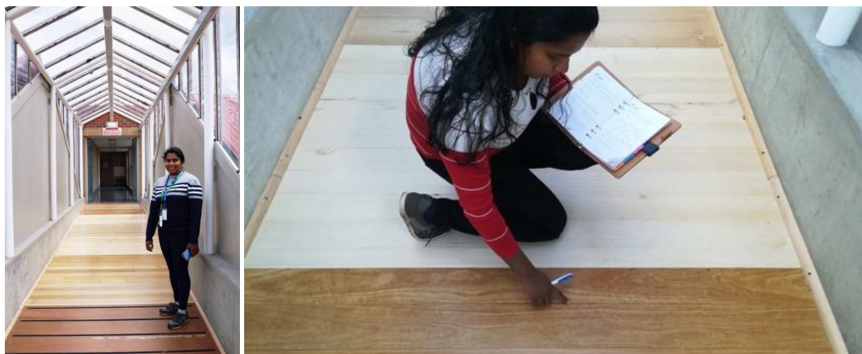
Figure 10: Traditional floor laid as a control
