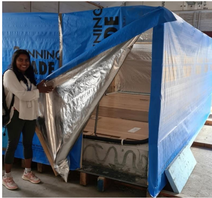
Figure 31: Protective enclosure around the floor
