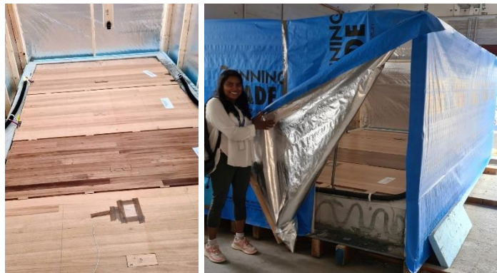
Figure 6: Completed floor and enclosure
