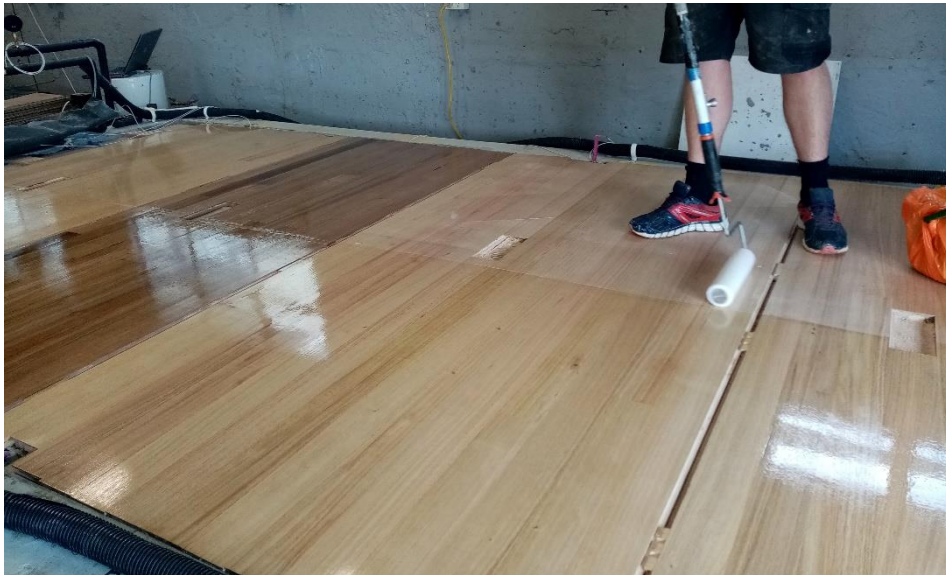
Figure 4: Finishing coat to the sanded flooring panels. Note the two floor finishes
