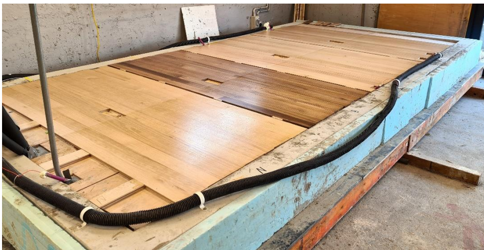
Figure 5: Completed flooring panels
