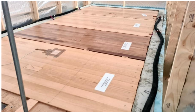
Figure 9: Floors during the heating trial
