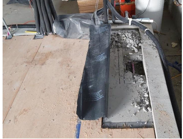
Figure 3: Repair to punctured water pipe
