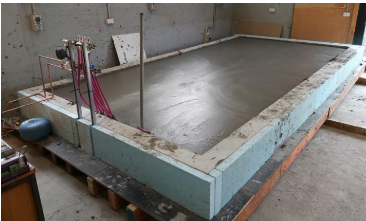
Figure 25: Topping to the heater slab
