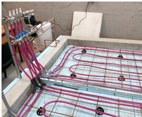
Figure 5: Base slab and hydronics
