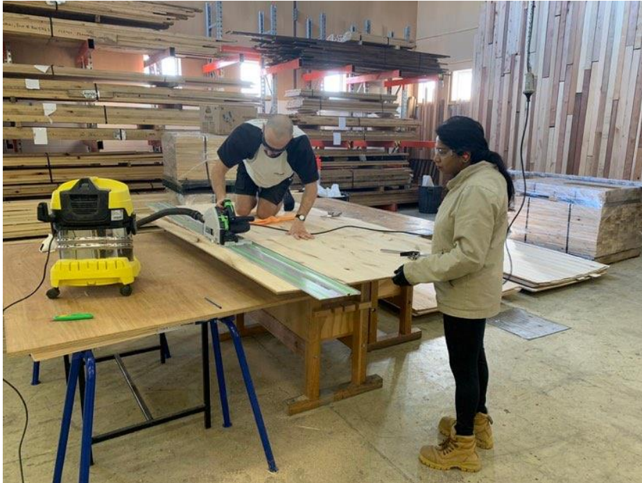
Figure 15: Ripping panels into single overlay lengths at CSAW workshop.
