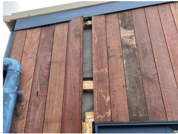
Board removed to relieve expansion pressure.
