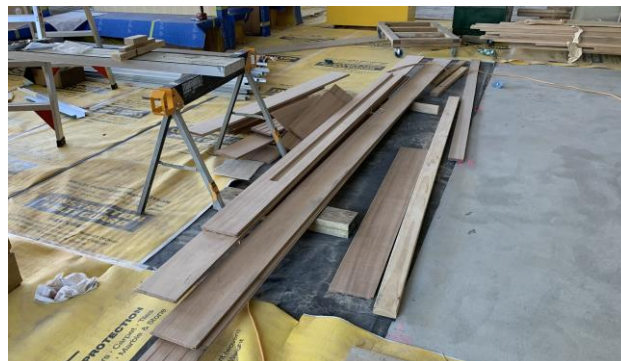
Figure 18: CZ7 construction – fitout
