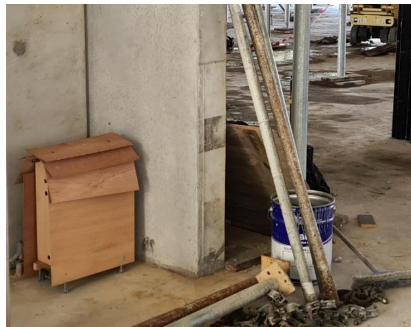
Figure 8: Static unit at a multistorey construction site at Launceston.
