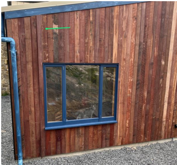
Figure 9: Expansion in vertical cladding on a south-facing wall
