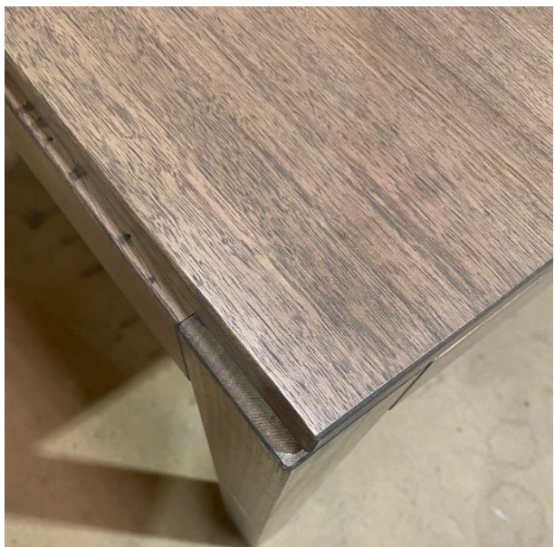
Figure 8: Shrinkage along a tabletop leading to an exposed rail edge
