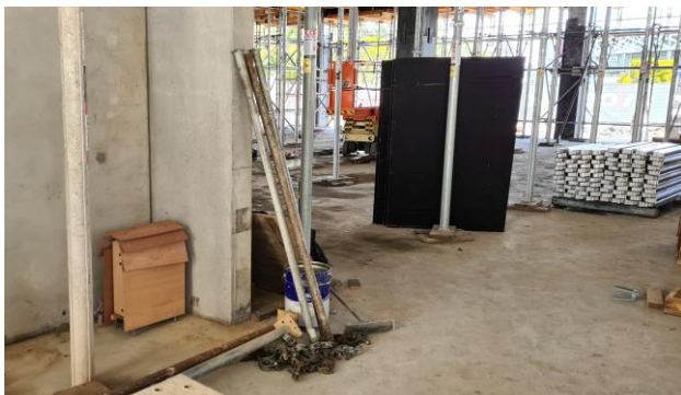
Figure 17: CZ7 construction – at frame stage
