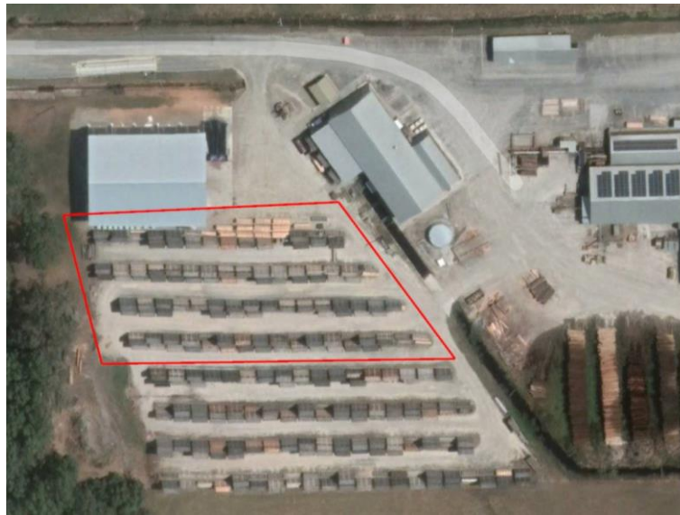
Figure 18: Drying area for the highly discoloured racks in Site 1a (east)
