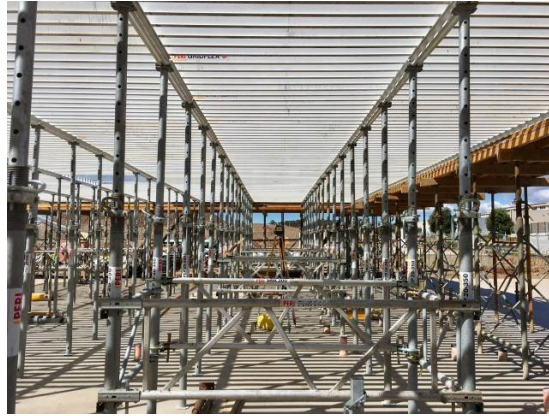
Figure A4: Gridflex bracing bays (Image credit: Perri)
