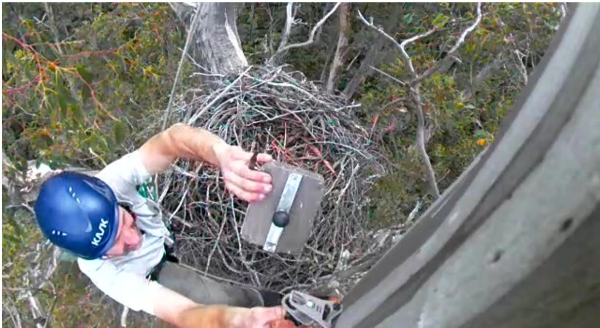
Figure 11: The sensors and cameras were installed by climbing the nest tree and securing them to the tree trunk above then nest with brackets featuring ball joints so the devices could be aimed directly down at the nest bowl.
