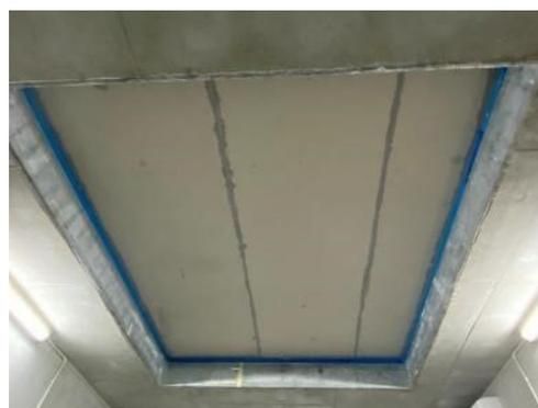
*Ceiling with Acoustic Sealant Treatment*
